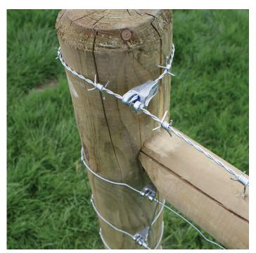
T-Clip 2 - Used to terminate barbed wire..
